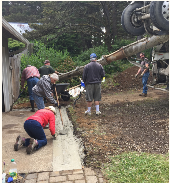
EXPERT CAREGIVERS AT WORK ON CONCRETE AROUND DRIVEWAY DRAIN
